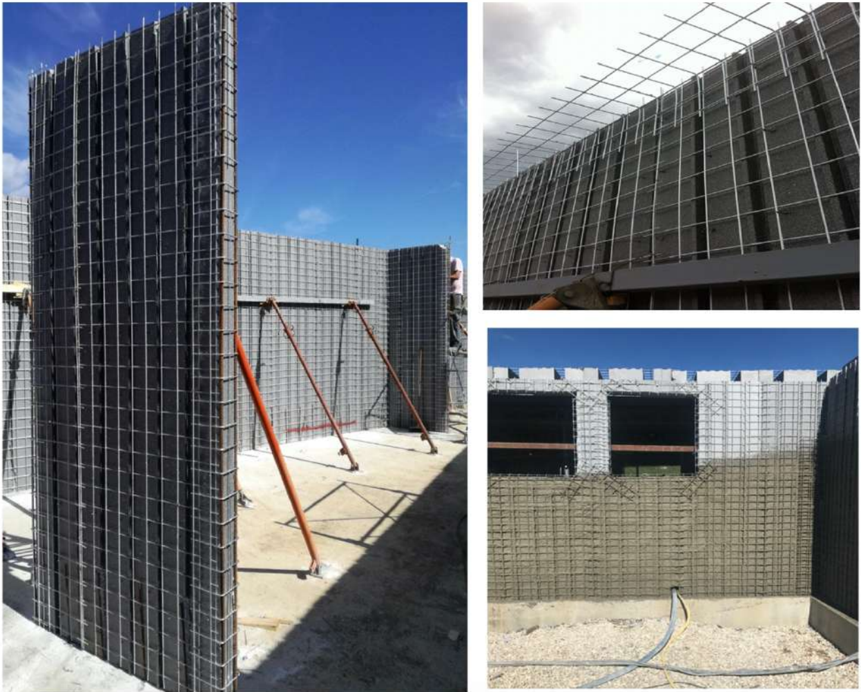
Figure 1. Production and mounting procedures for sprayed-in-situ RC sandwich panels
