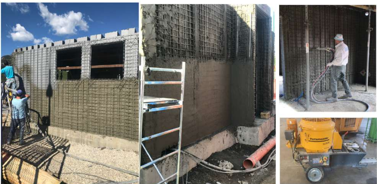
Figure 2. Spraying technique procedure
