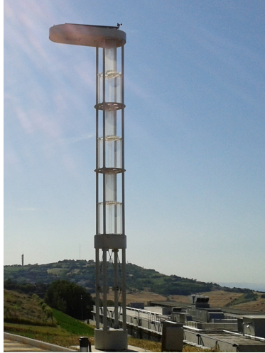
Figure 1: The UNIVPM prototype of the experimental street lamp powered by renewable sources.
