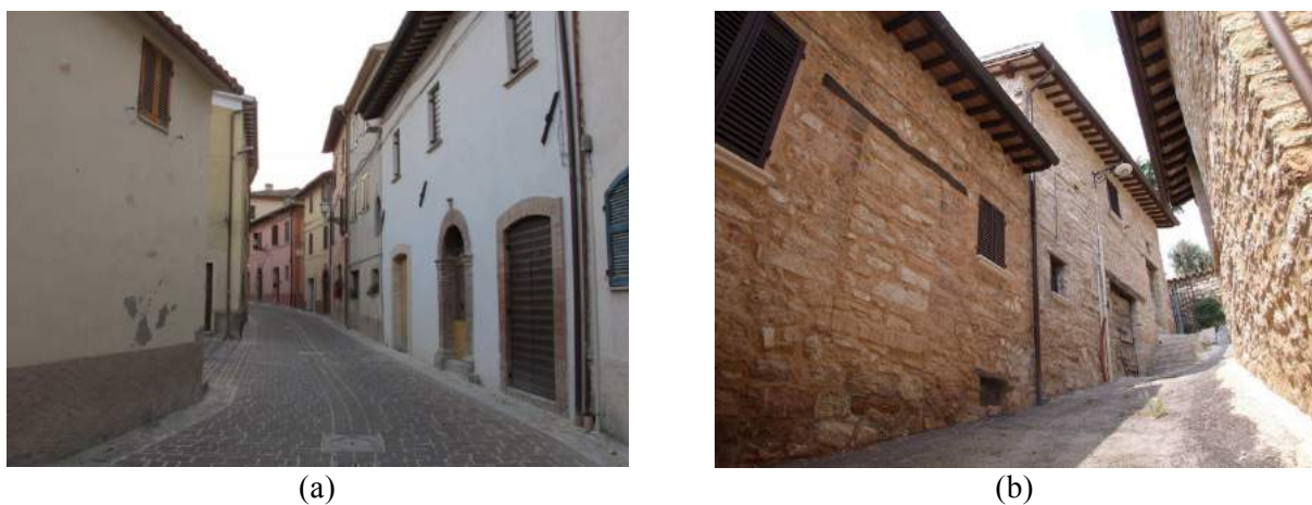
583 Figure 8. Building conformation: a) vertical configuration; b) structural heterogeneities. 584 585 586 587 588 589 590
