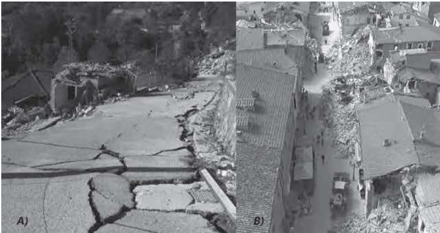
1223 1224 Figure 2 Urban scenario damages in the Central Italy seismic sequence in 2016: A) street pavement cracking due to unstable slopes 1225 and landslides-induced effects (Intrinsic vulnerability); B) an aerial view of Amatrice (RI, Italy) main street, that is partially blocked by 1226 ruins formation provoked by buildings collapse; debris impeded rescuers' interventions (Extrinsic vulnerability). Video frames by Corpo 1227 Nazionale dei Vigili del Fuoco http://www.vigilfuoco.tv/ (last access 2018/04/17). 1228 1229
