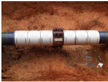
(a) Crack arrestor installed.
