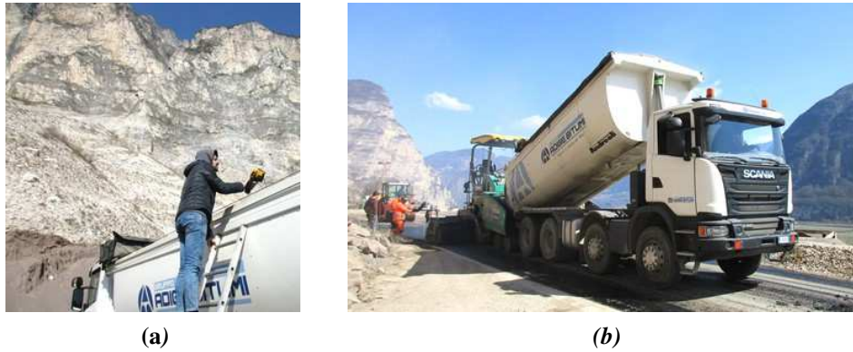
Figure 66 - Pictures from the field investigation: (a) temperature measurement; (b) HMA delivery to the paver.
