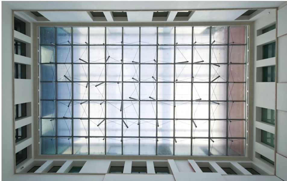
Figure 2.10. Roof of the Archeological Museum of R. Calabria.
