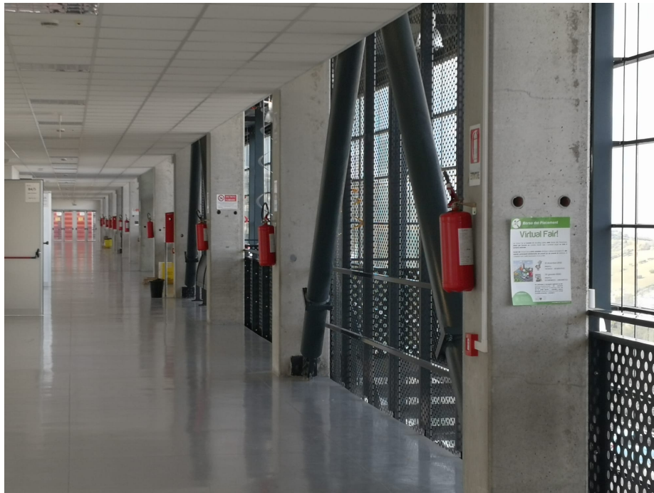
Figure 5.6: First floor corridor showing the longitudinal development.
