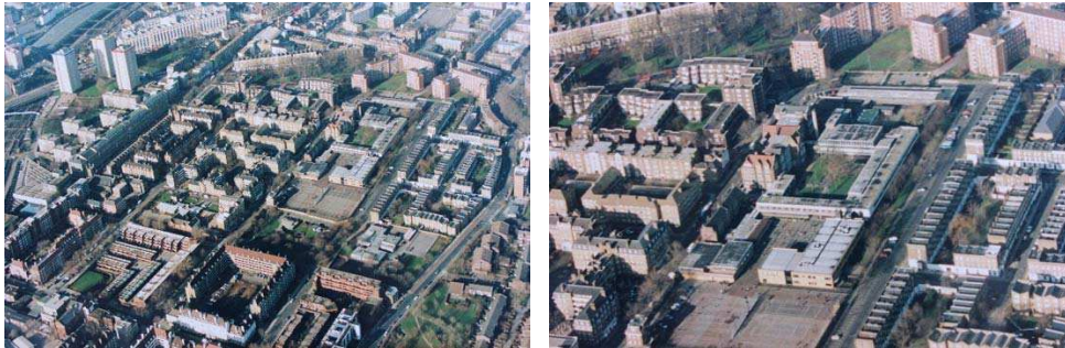
Fig. 4-46 Aerial view of Chalton street and Somers Town area and zoom on South Camden Community School before the renovation and conversion in Regent High School (© photos by Regent High School Archive).
