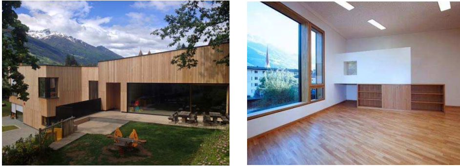
Fig. 2-25 Kindergarten at Silandro (Bolzano), Italy. Building by Christian Kapeller and Stephan Marx. (Photo ©Rene Riller and Christian Kapeller).
