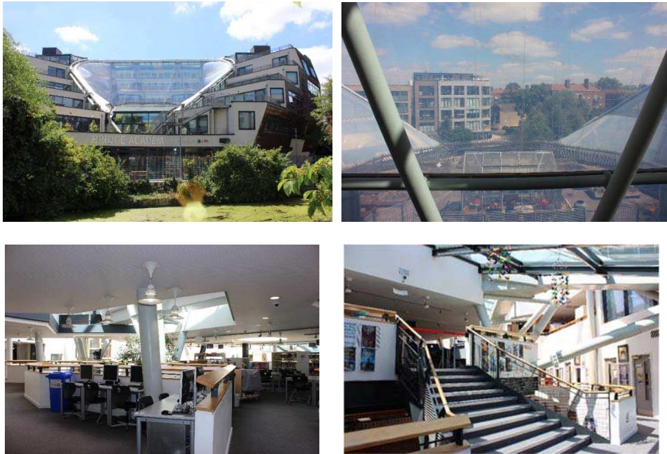
Fig. 4-77 External and internal views. Details of the roof in ETFE.
