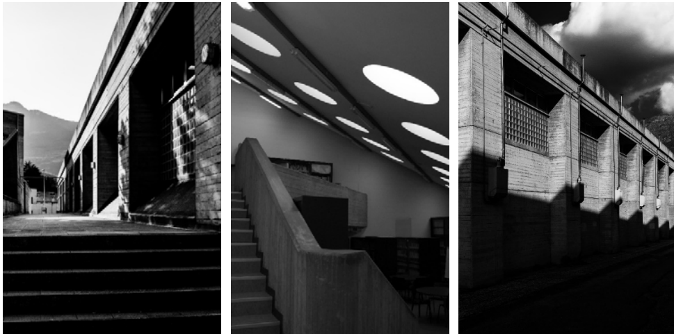
Fig. 2-21 Technical institute for surveyors "Bovara" a Lecco, Italy. Building by Enrico Mantero, 1970 (©Francesco Pavan)
