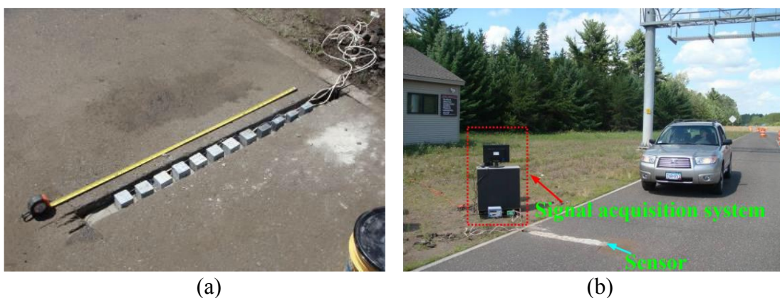
Figure 2.9. Self-sensing system for traffic monitoring: a) Placement of the cement-based sensor array; b) Overview of the system [80]
