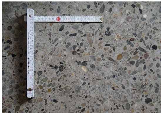
Figure 2.2. Traditional concrete surface. Aggregates are distinguishable from the cement matrix
