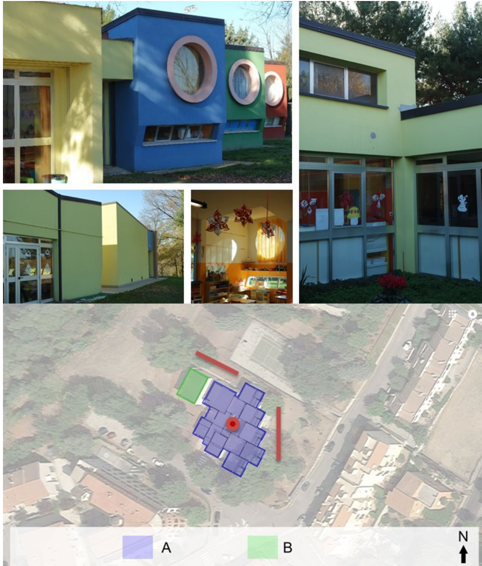
Figure 4.23 Analysed buildings of the third school complex.
