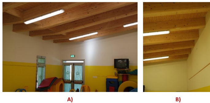
Figure 4.25 Photographic views of Building B.
