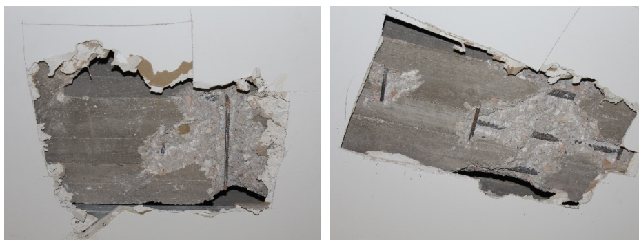
Figure 4.12 Inspection to verify not complying steel reinforcements of beams (Ripe).
