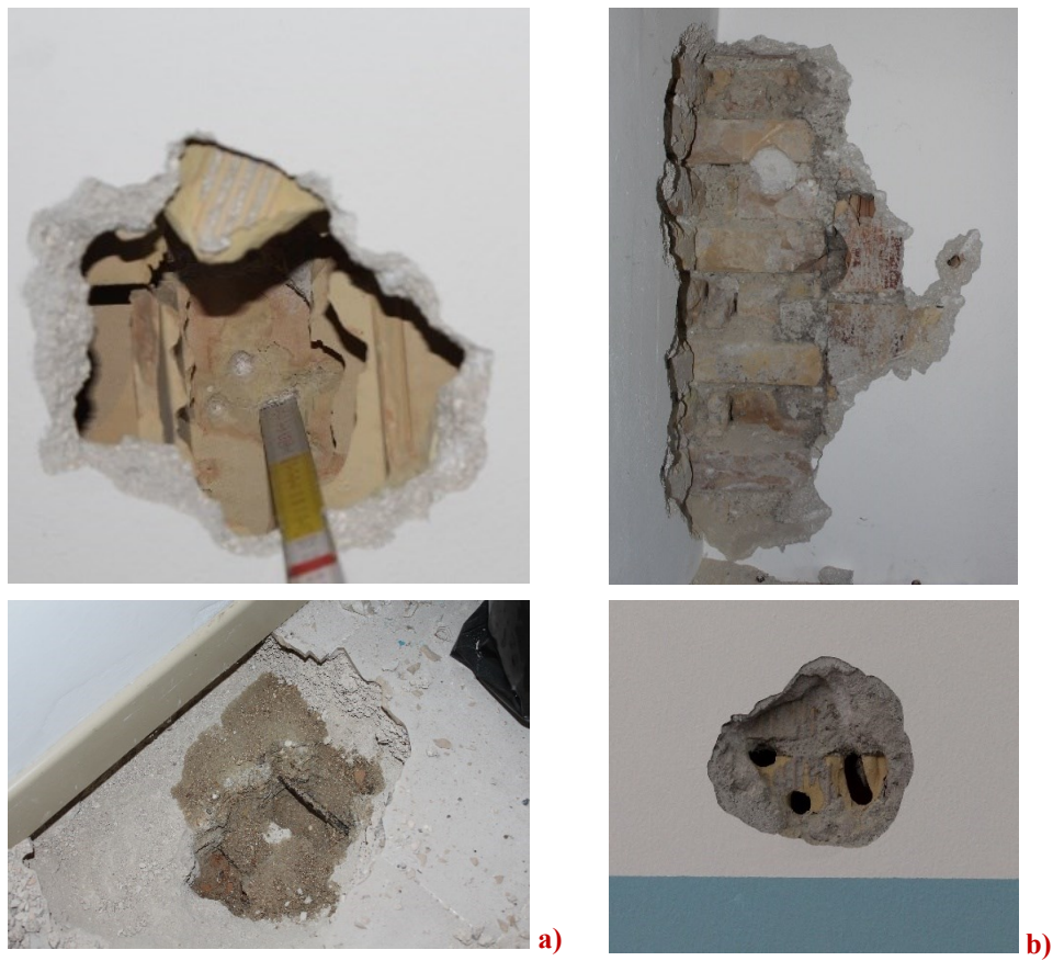
Figure 4.11 Inspection holes in floors (a) and peripheral walls (b) (Castel Colonna).
