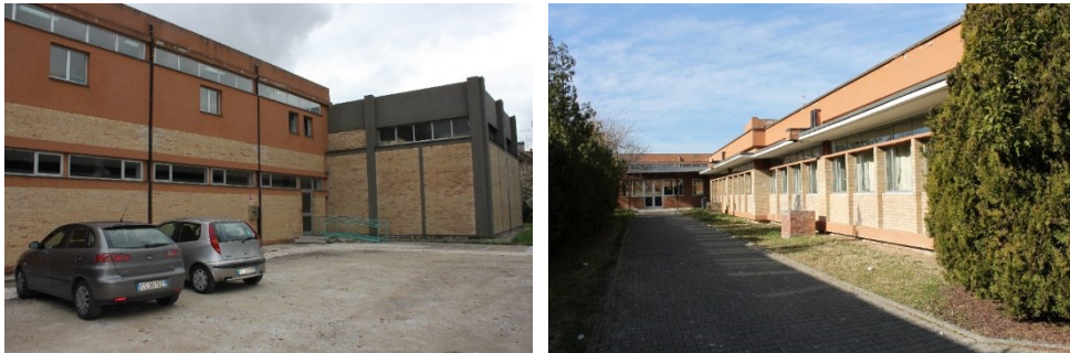
Figure 1.4 A RC school complex in the municipality of Trecastelli built in 70s.
