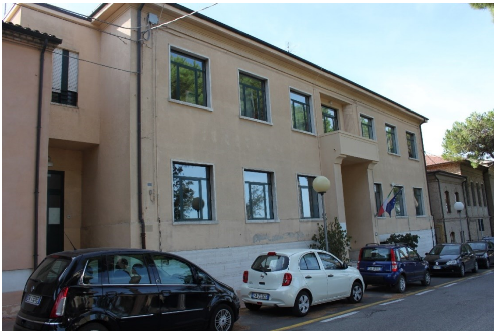
Figure 1.3 A masonry school building in the municipality of Trecastelli, later expanded with other structurally independent buildings.
