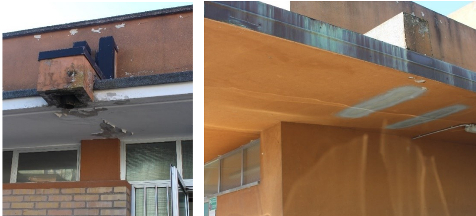
Figure 3.5 Strongly protruding cornices and shelters (Ripe).
