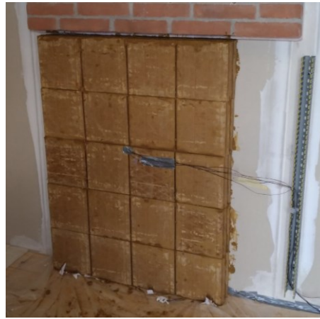
Figure 3.7: Earth blocks masonry panel built in the internal southbound wall.
