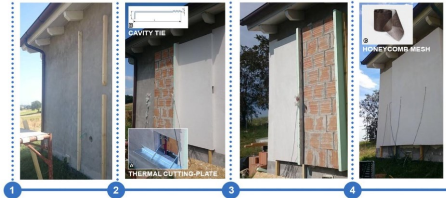
Figure 3.5: Construction phases of the ventilated prototypes.
