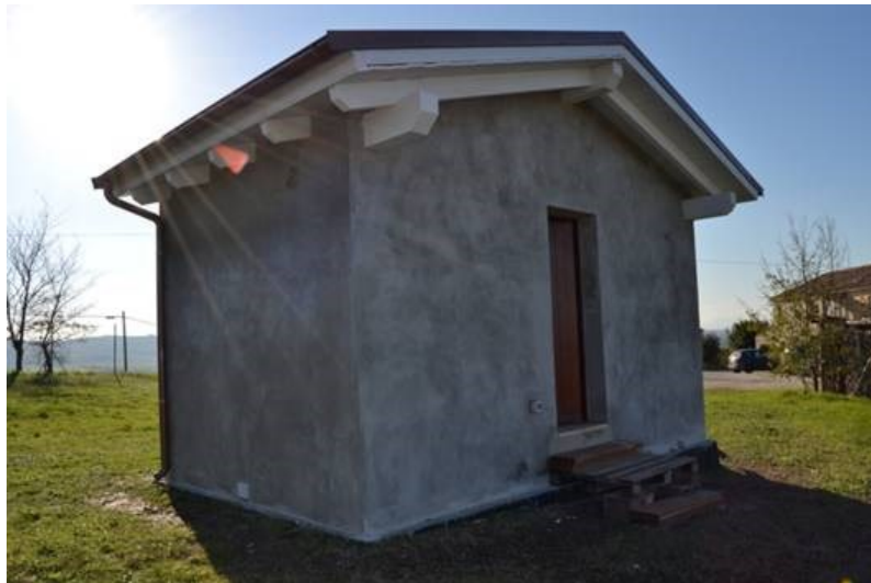
Figure 3.1: External view of the mock-up.
