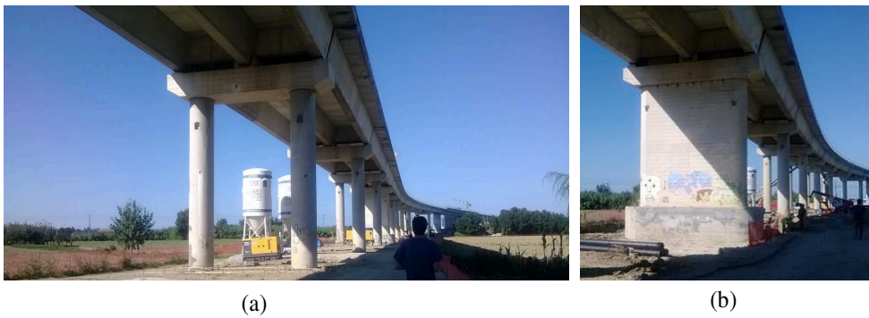
Figure 3.3 (a) Cross section of the viaduct and column bent pier, (b) wall pier
