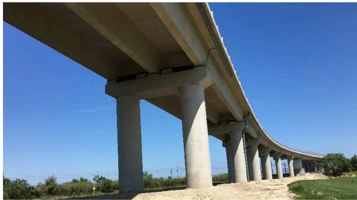
Figure 4.21 “Chiaravalle viaduct” view after retrofitting works
