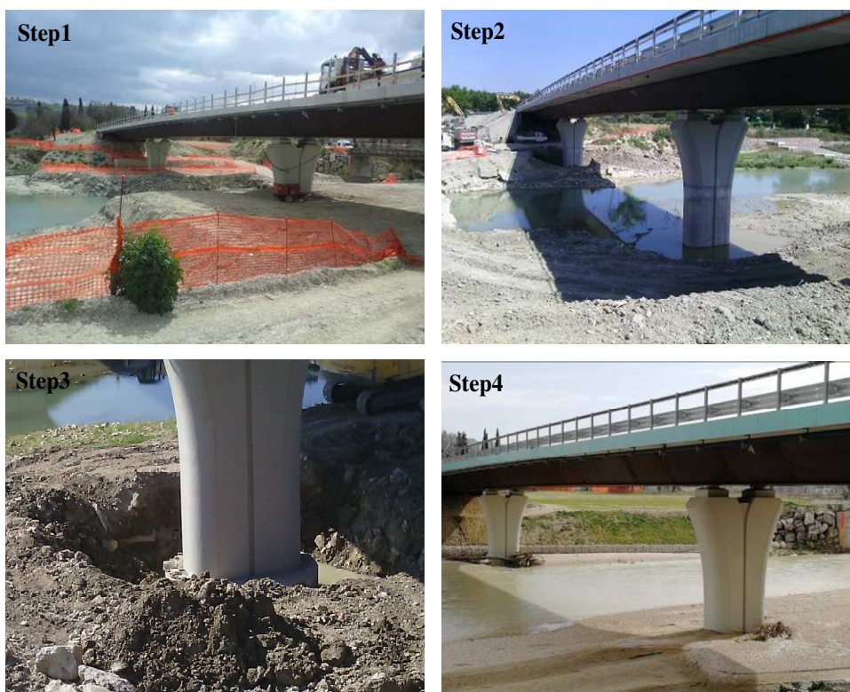
Figure 3.13 Images of the “Cesano bridge” piers at different construction steps
