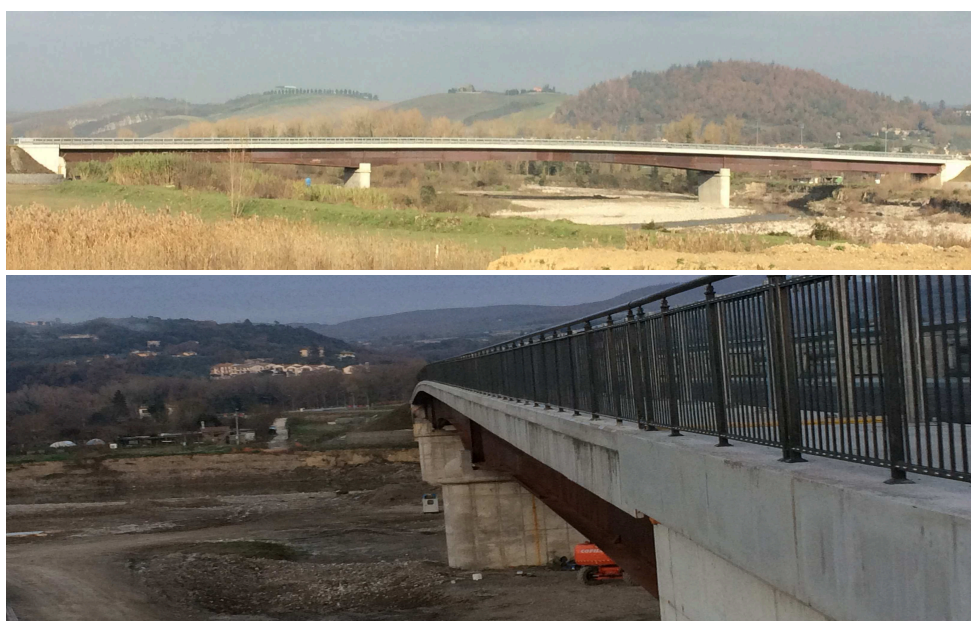
Figure 3.9 Lateral views of “Paglia bridge”, Orvieto
