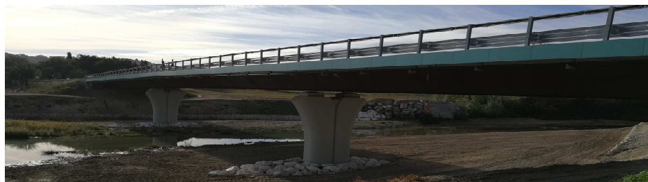
Figure 3.12 Global view of “Cesano bridge”
