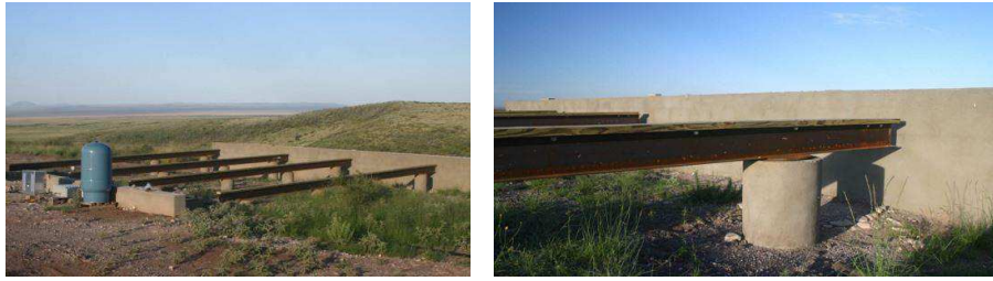
Figure 3.8: Preparation of foundation for Prefabricated houses [29]
