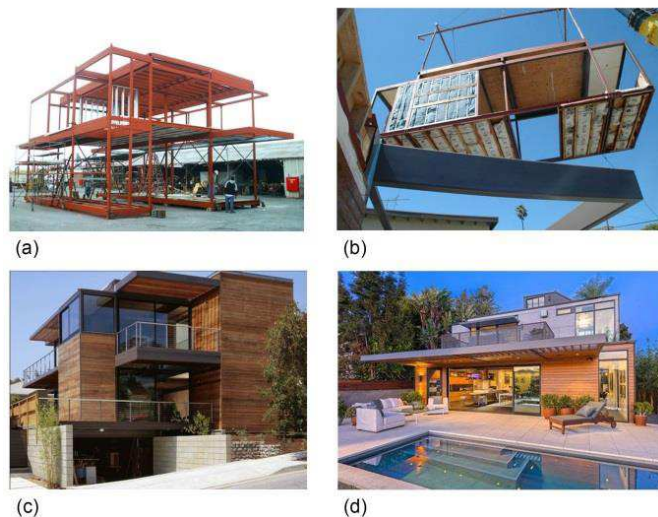
Figure 2.5: Living home series, US, (a) construction phase, (b) Installation phase, (c) Completed project, (d) Custom Ray, Designed by Ray Kappe, US [30]
