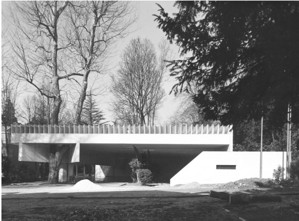
Fig.165 – Nordic Pavilion by Sverre Fehn at the Venice Biennale. Source: Photo Ferruzzi, The National museum of Art, Architecture and Design, Oslo..
