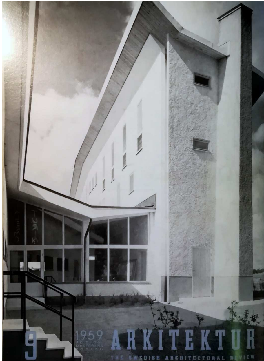
Fig.157 – The Italian Institute of Culture on the cover of Arkitektur (1959) Source: Arkitektur 9 (1959).
