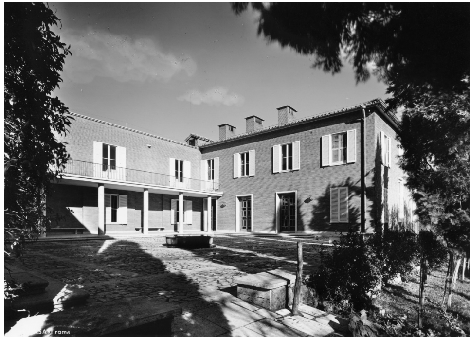
Fig.85-86 – Swedish Institute: West facade ( above ) and East court ( below ). Source: Ark Des, Stockholm. Photo by Vasari (Rome), ID. ARKM.1984-102-1320 ( above ) and ID. ARKM.1984-102-1324 ( below ).
