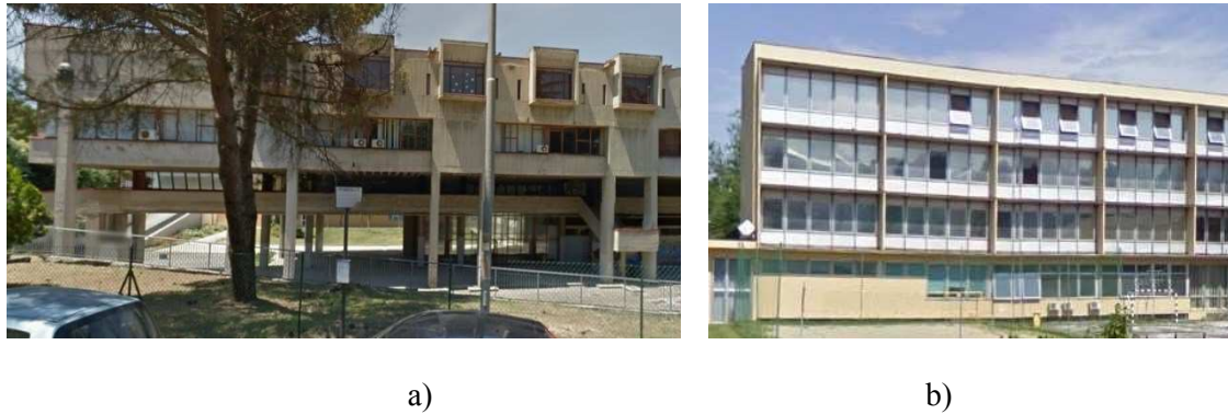
Figure 4.17. Arcades at the ground floor (a), short columns on the façade (b)
