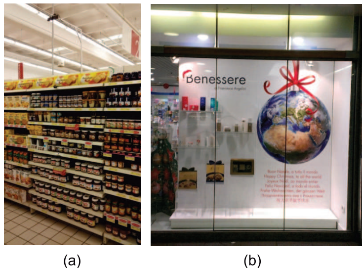
Figure 3.7: Details of Shopper Analytics roll out phase. (a) Camera installed above shelves of Ferrero's products. (b) Camera installed on Angelini's pharmacy showcases.
