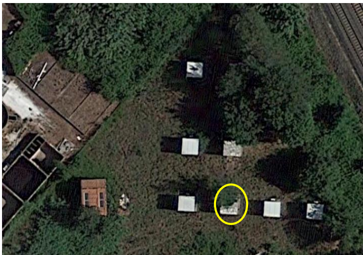
Figure 143. Site map. The used pilot test room is circled, Google Maps.
