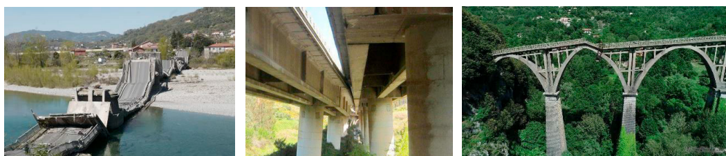
Fig. 1. A) Albiano Magra bridge; b) Himera Viaduct, c) Serra railway viaduct.
