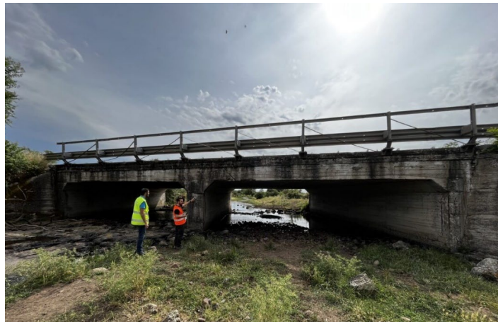
Figure 23. Photo of the concrete frame bridge.
