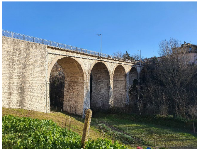
Figure 29. Photo of the concrete arch bridge.
