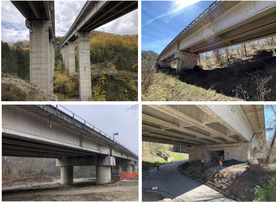
Figure 35. Some photos of the Prestressed RC bridges from the set.
