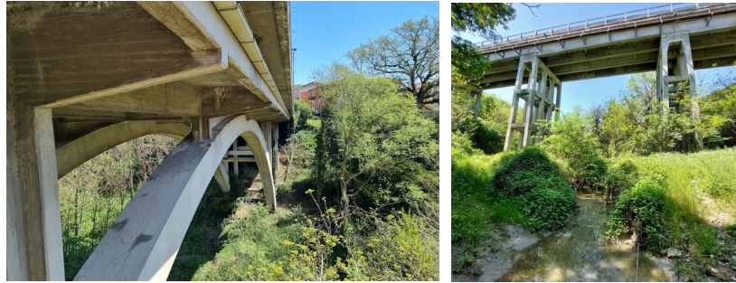
Figure 31. Concrete bridges with variable beam cross-sections.
