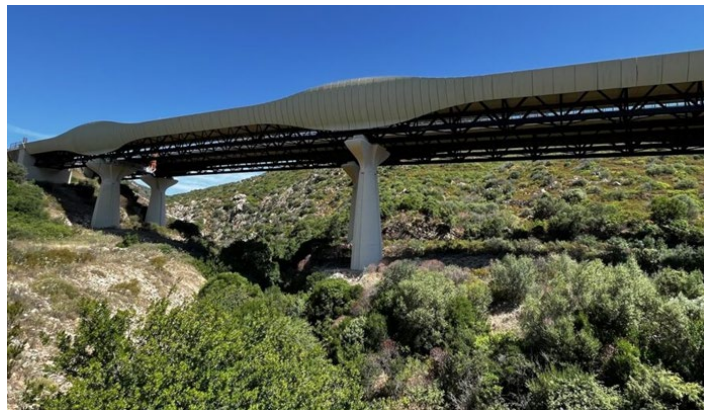
Figure 19. Panoramic photo of the steel composite bridge.
