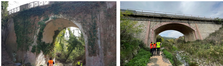
Figure 15. Photos of the two masonry arch bridges.
