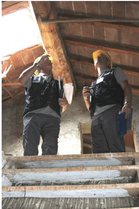
Figure B1: Example of the assessment of the damage in a building in damaged zone. Source: Dolce and Di Bucci (2014, p. 2244)
