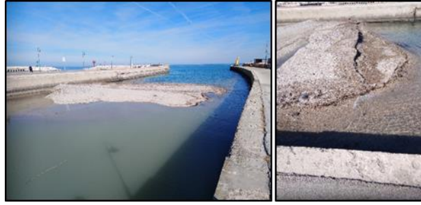
Fig. 1. Images of the bar formed inside the mouth of the Misa River.
