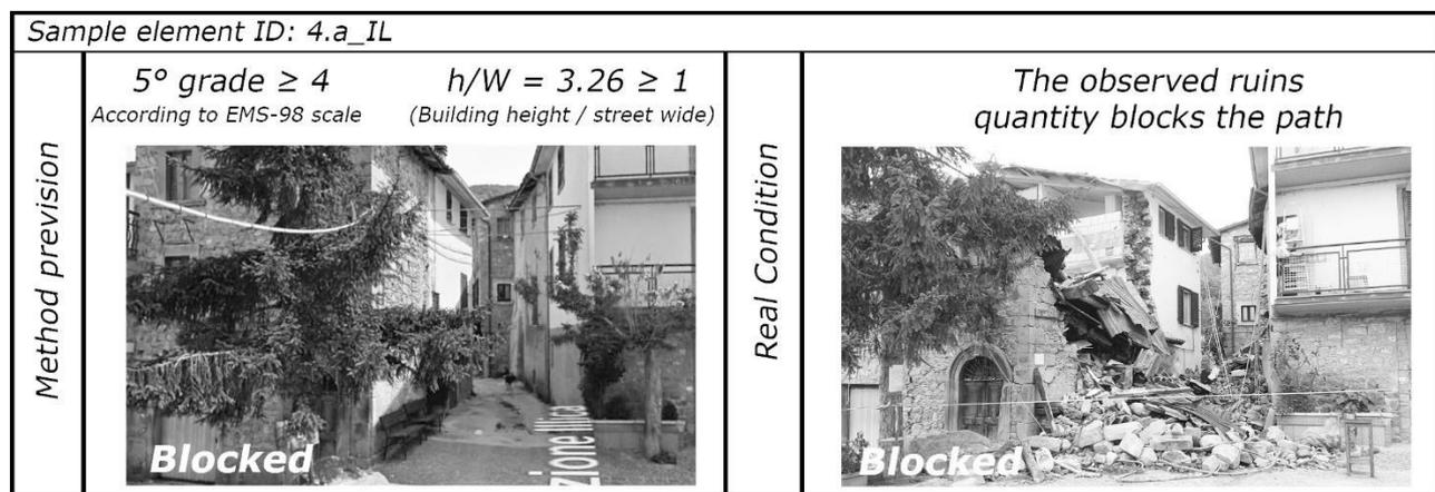
**Figure 2** Comparison between the *Observed* macroseismic damages-based approach prevision and real conditions of path blockage for a building in the sample (Element ID code: 4.a\_IL in **Appendix B**): the path is effectively blocked because the observed damage is higher than the 4<sup>th</sup> grade and the ratio between building height and street width is higher than 1.
