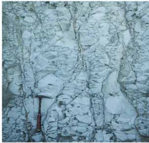
Figure 13. Complex fracturing of the Schlier formation with rugged surfaces and complex shapes of the blocks.
