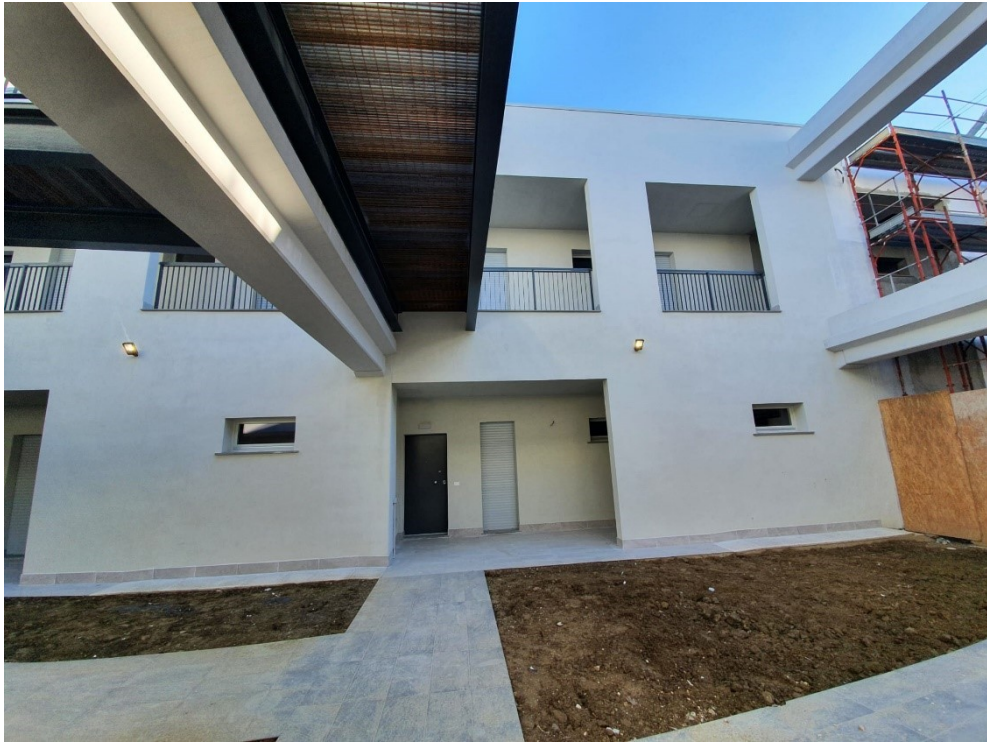
Figure 31: Walkways of the inner courtyard at ground floor level
