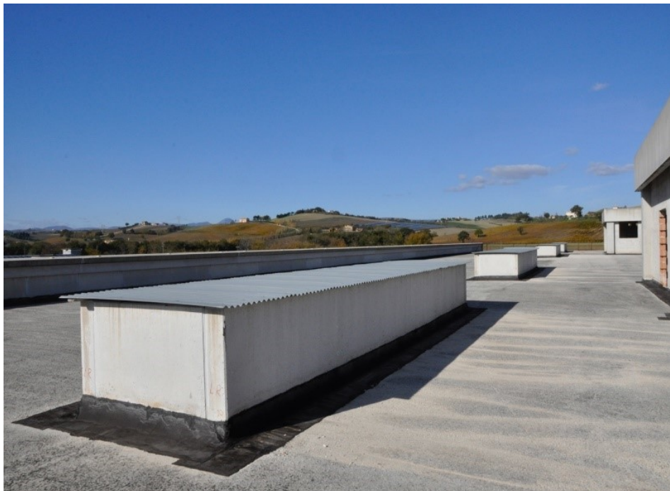
Figure 27: Roof original appearance
