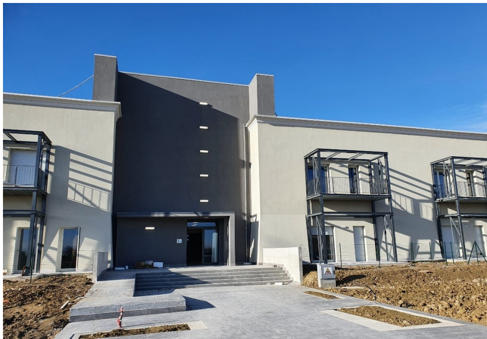
Figure 21: Building after renovation
