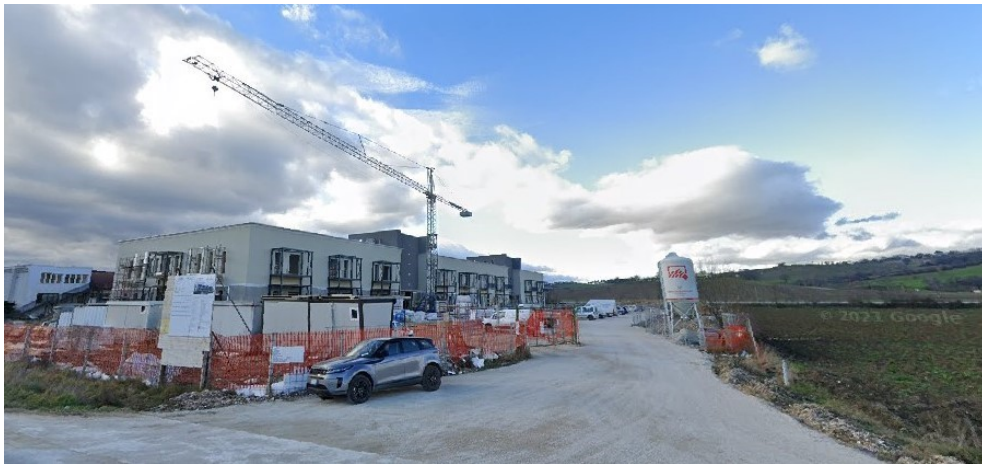
Figure 62: View of the renovation works
