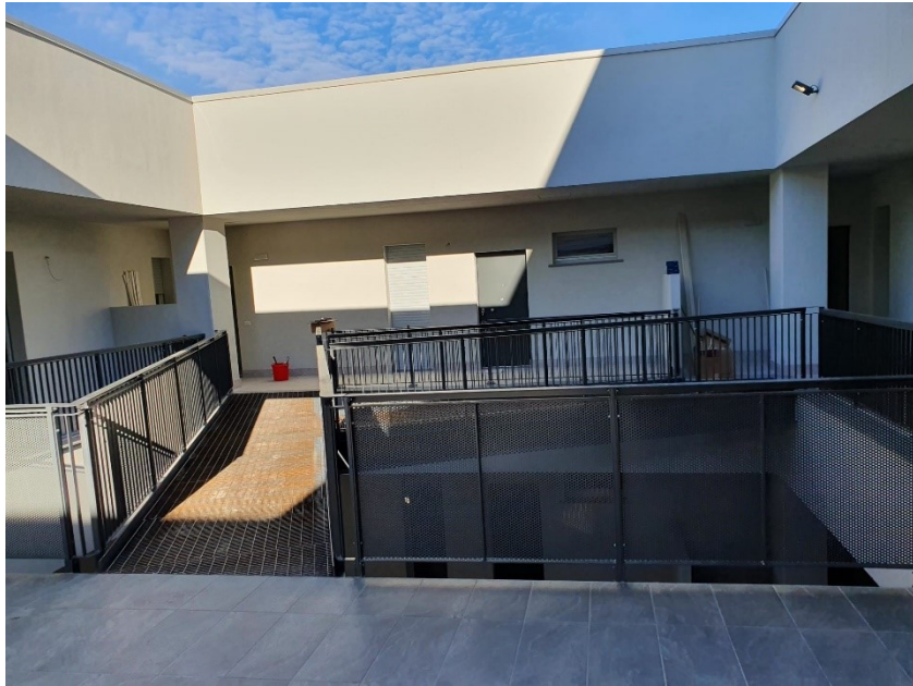
Figure 30: Walkways of the inner courtyard at first floor level
