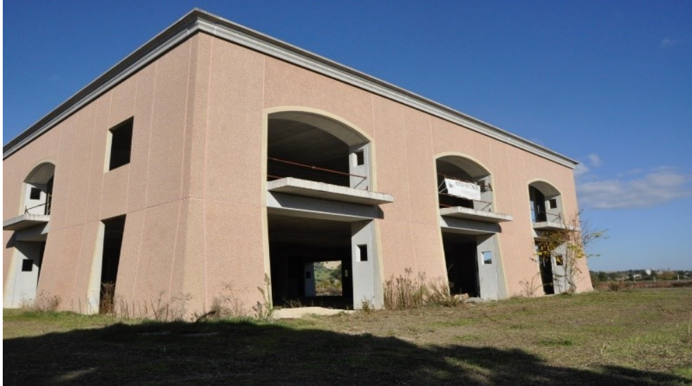
Figure 22: Building original appearance
