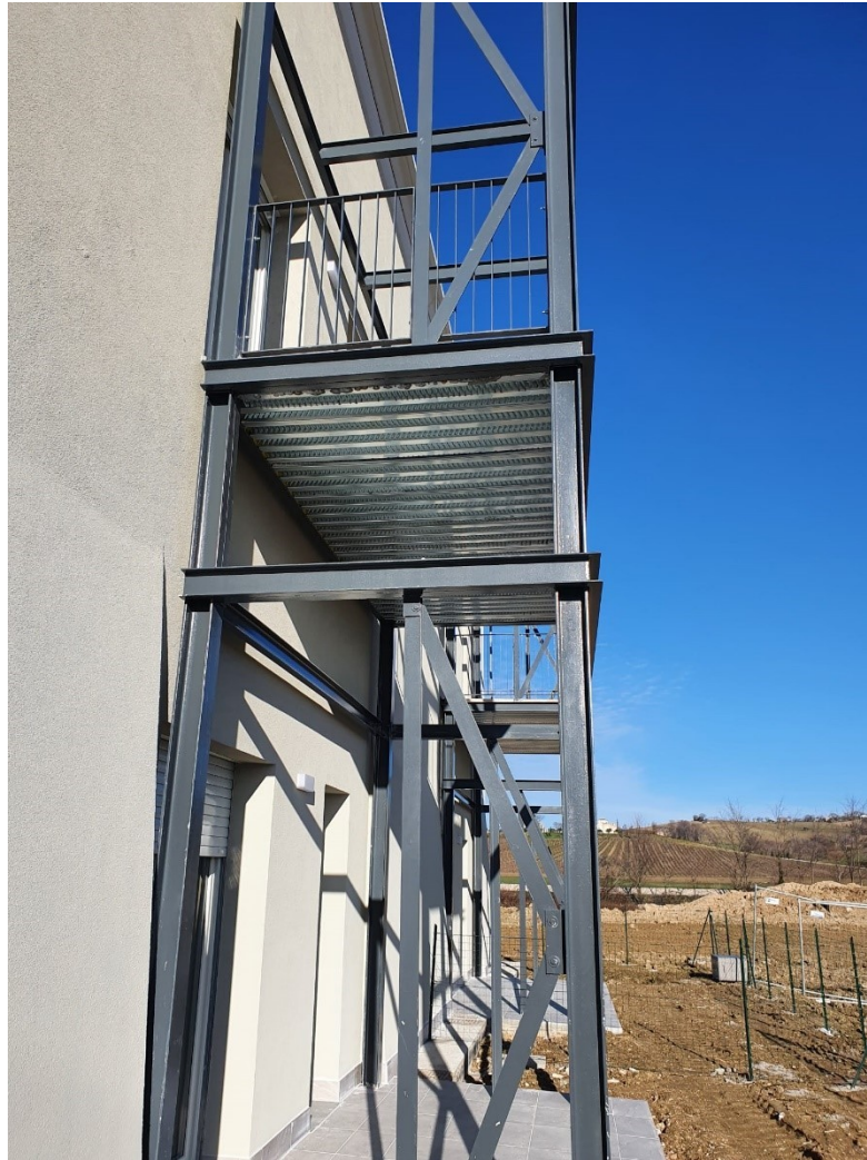
Figure 28: Self-supporting terrace
