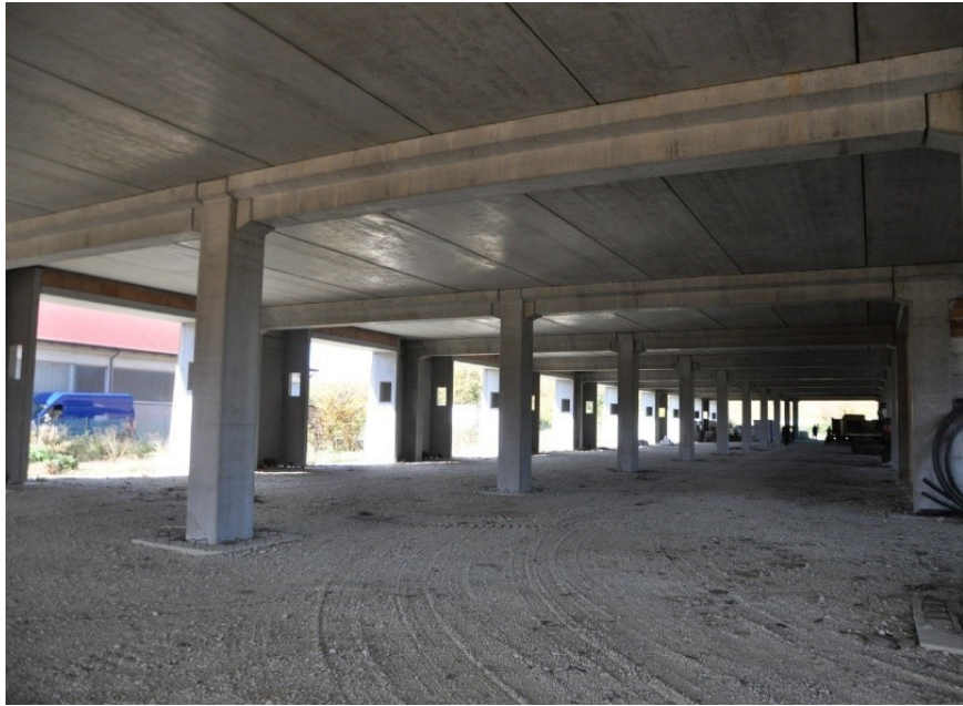
Figure 24: Ground floor at the beginning of the renovation works
