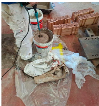
Figure 2. Preparation of Porotherm special mortar.
