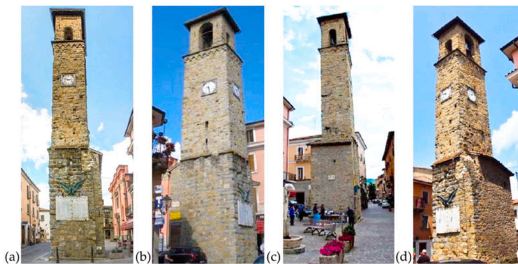
Fig. 3. – View of the Civic Tower South (a), West (b), North (c) and East façade (d).
