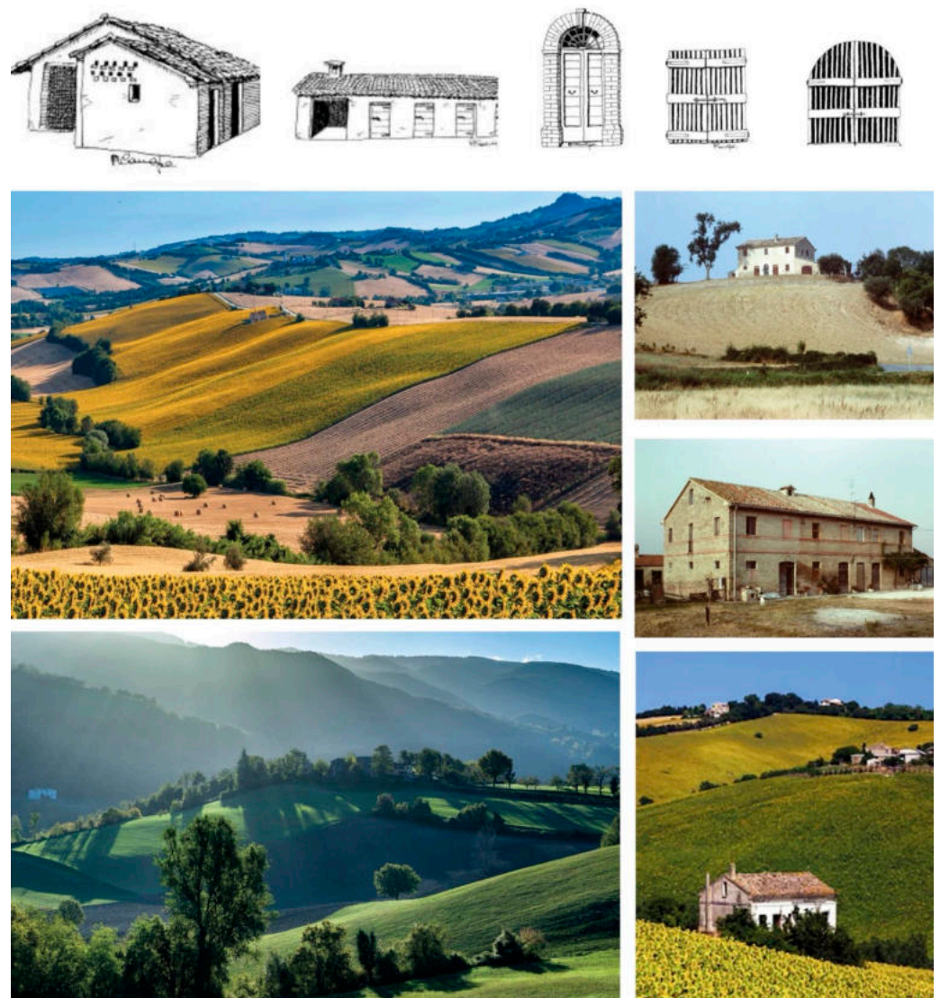
Figure 5. Traditional Marche farmhouses: typological features, architectural components, and integration within the hilly landscape. Bottom right: mid-slope farmhouse in Cesano di Senigallia. Top right: hilltop farmhouse with internal staircase in Castelvecchio di Monteporzio, Pesaro.
