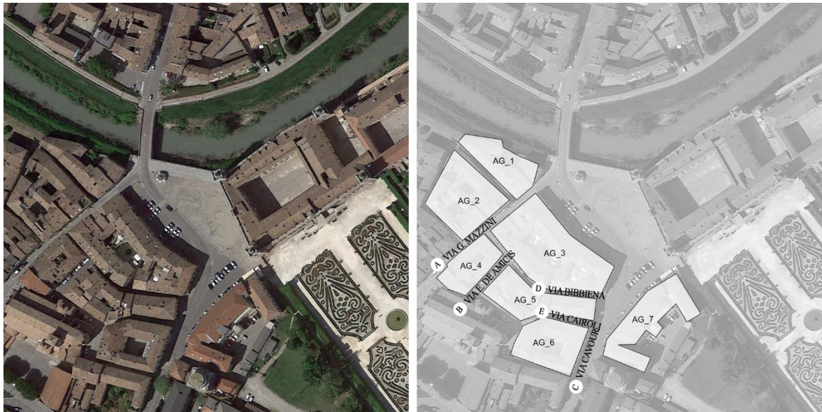
Figure 77: POS “Piazza Garibaldi” area in Colorno – streets and building blocks included in the case study.
