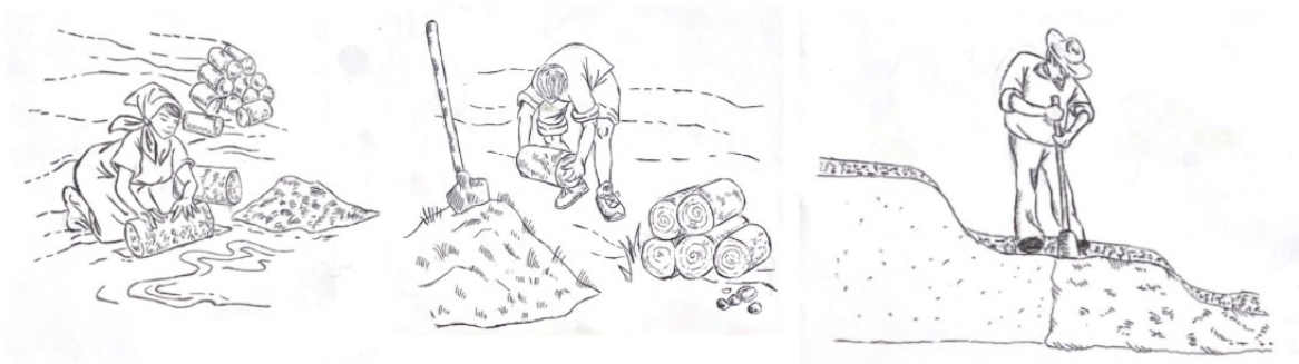
Figure 69: Three main phases for the construction of Cob masonry buildings [61].
