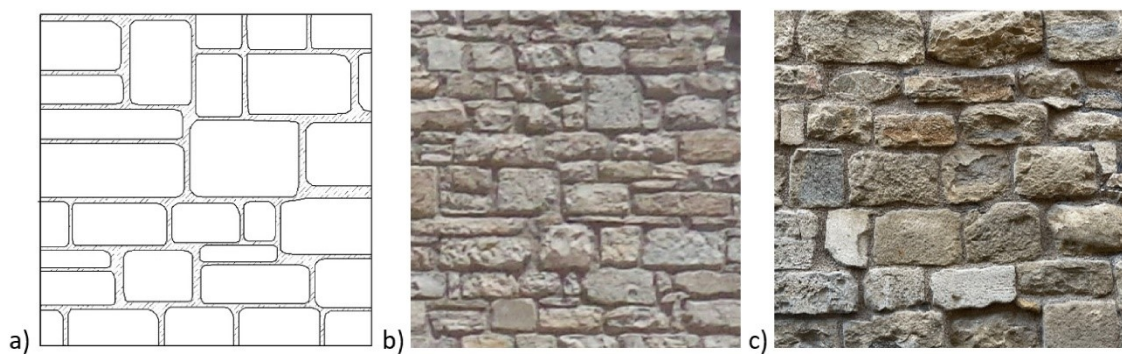
Figure 62: Roughly cut stone with good texture (M3) – a) Graphic reconstruction of the wall texture type (1mx1m); b) Wall façade example, photo taken in Castelsantangelo sul Nera (MC); c) Wall façade example, photo taken in Cingoli (MC).
