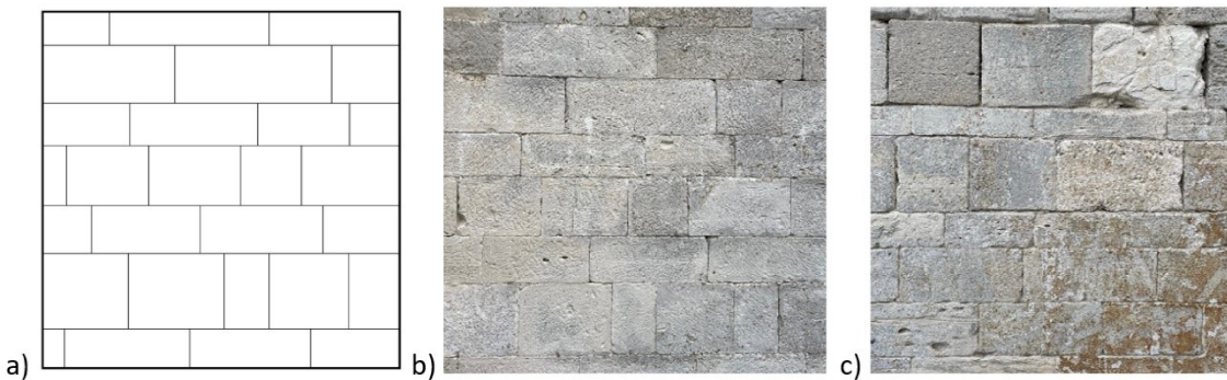
Figure 65: Stone blocks squared (M6) – a) Graphic reconstruction of the wall texture type (1m x 1m); b) Wall façade example, photo taken in Cingoli (MC); c) Wall façade example, photo taken in Muccia (MC).
