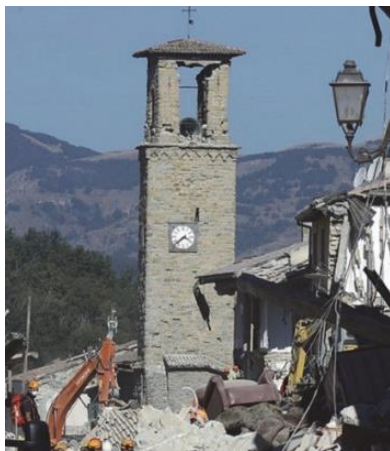
Figure 8. Belltower in Amatrice, damaged by the earthquake in 2016 (unconfined tower)
