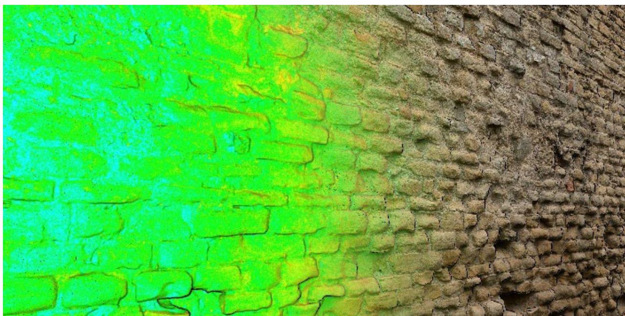
Figure 2. Detail of the masonry texture reconstructed in 3D through laser scanning.
