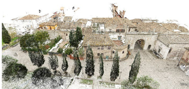
Figure 3. View of a portion of the point cloud of the Walls of Fano, derived from the integration of TLS and UAV photogrammetry.
