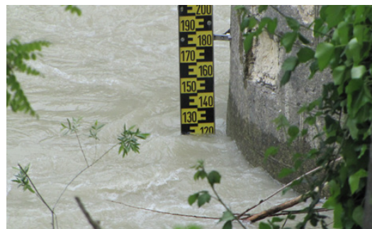
Figure 2. Example of hydrometric rod installed by the Civil Protection in the municipality of Acqualagna (PU), Candigliano basin. The hydrometric rod (also called staff gauge [5]) is made of anodized aluminum with anti-corrosion treatment to resist even environments with contaminants and abrasions. The high color iridescent effects allow excellent visibility of scale even at a considerable distance and in any application (concrete, bricks, soil, etc.).
