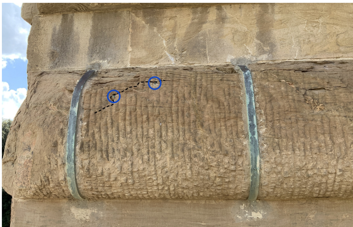
Figure 16. Florence, Pitti Palace, Cortile dell'Ammannati. Critical stone ashlars due to previous interventions and material discontinuities in the test area (Photos by Chiara Mariotti and Alessandro Ceppetelli 2022).
