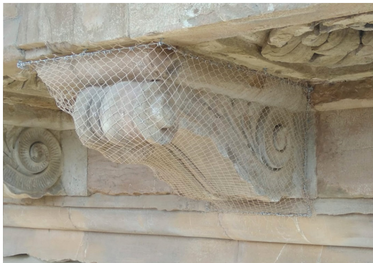
Figure 4. Florence, Pitti Palace, Cortile dell'Ammannati. Temporary fall protection systems made of nylon nets, installed on the façades during the 2018-19 monitoring campaigns (Photos by Stefano Landi and Andrea Bonaccorso 2019).
