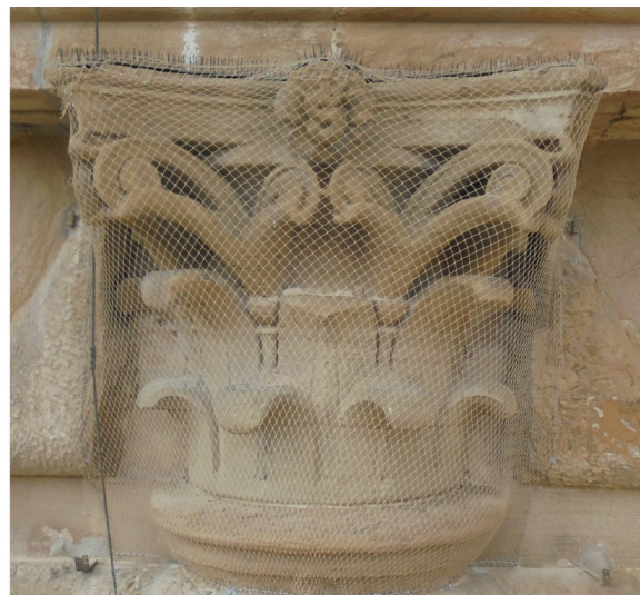
Figure 4. Florence, Pitti Palace, Cortile dell'Ammannati. Temporary fall protection systems made of nylon nets, installed on the façades during the 2018-19 monitoring campaigns (Photos by Stefano Landi and Andrea Bonaccorso 2019).
