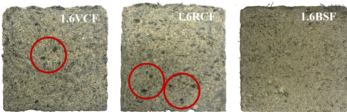
306 307 Fig. 6. Section of 1.6VCF and 1.6RCF specimens, where the agglomerated CFs clumps are clearly 308 visible, which cause air voids within the composite (red circle). Section of 1.6BSF shows a more 309 uniform structure. 310
