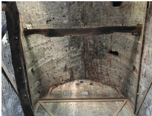
Figure 6.10: Tower masonry conditions
