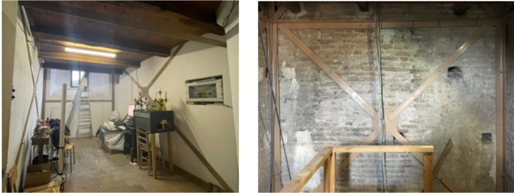
Figure 6.9: Tower safety intervention (2018)
