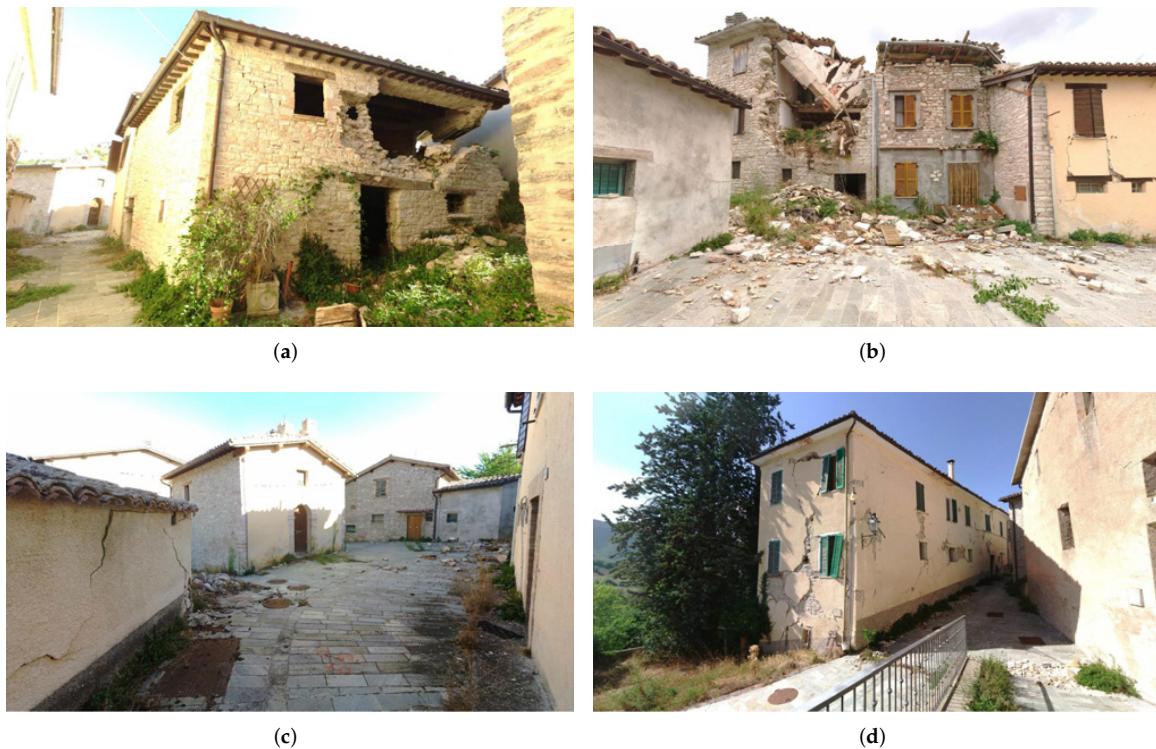
Figure 3. Damaged buildings in Gabbiano (Pieve Torina, Italy) on which is possible to observe different typologies of collapse. (a) Example of collapses stone Façade, (b) example of roof collapsed in stone buildings, (c) example of small urban area with cracks and (d) example of more recent building with cracks.
