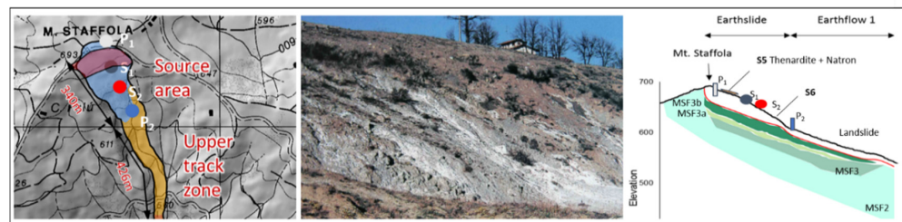
Figure 3. On the right, detail of the groundwater monitoring points in the source and earthslide1 zones (S1 and S2: springs; P1 and P2: piezometers) together with the area in which the thick white crusts (in purple) outcrop. In the middle, a photo taken in August 2015 in which the white powder is clearly visible together with the spring S2. Simplified geological cross section of the source and earthslide1 zone along with the groundwater monitoring points (P1, P2, S1, and S2) and soil samples S5 and S6.
