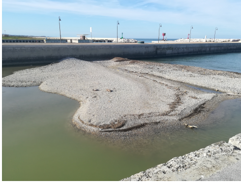
Figure 1.1: Image of the bar formed inside the mouth of the Misa River.
