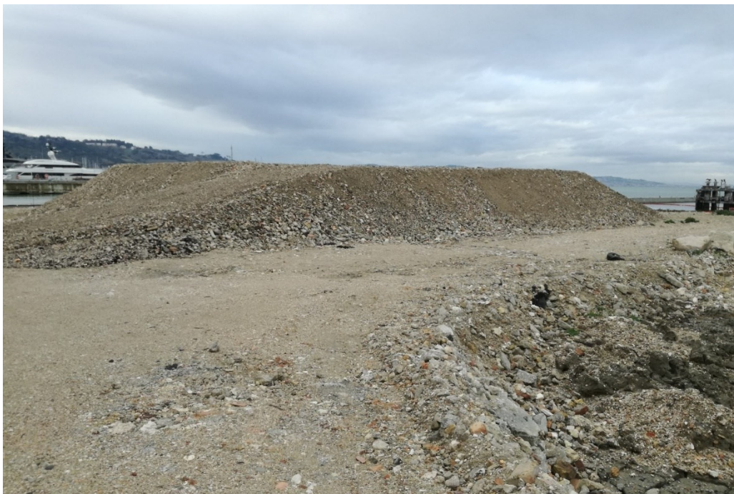
Figure 5.35. The finished embankment.
