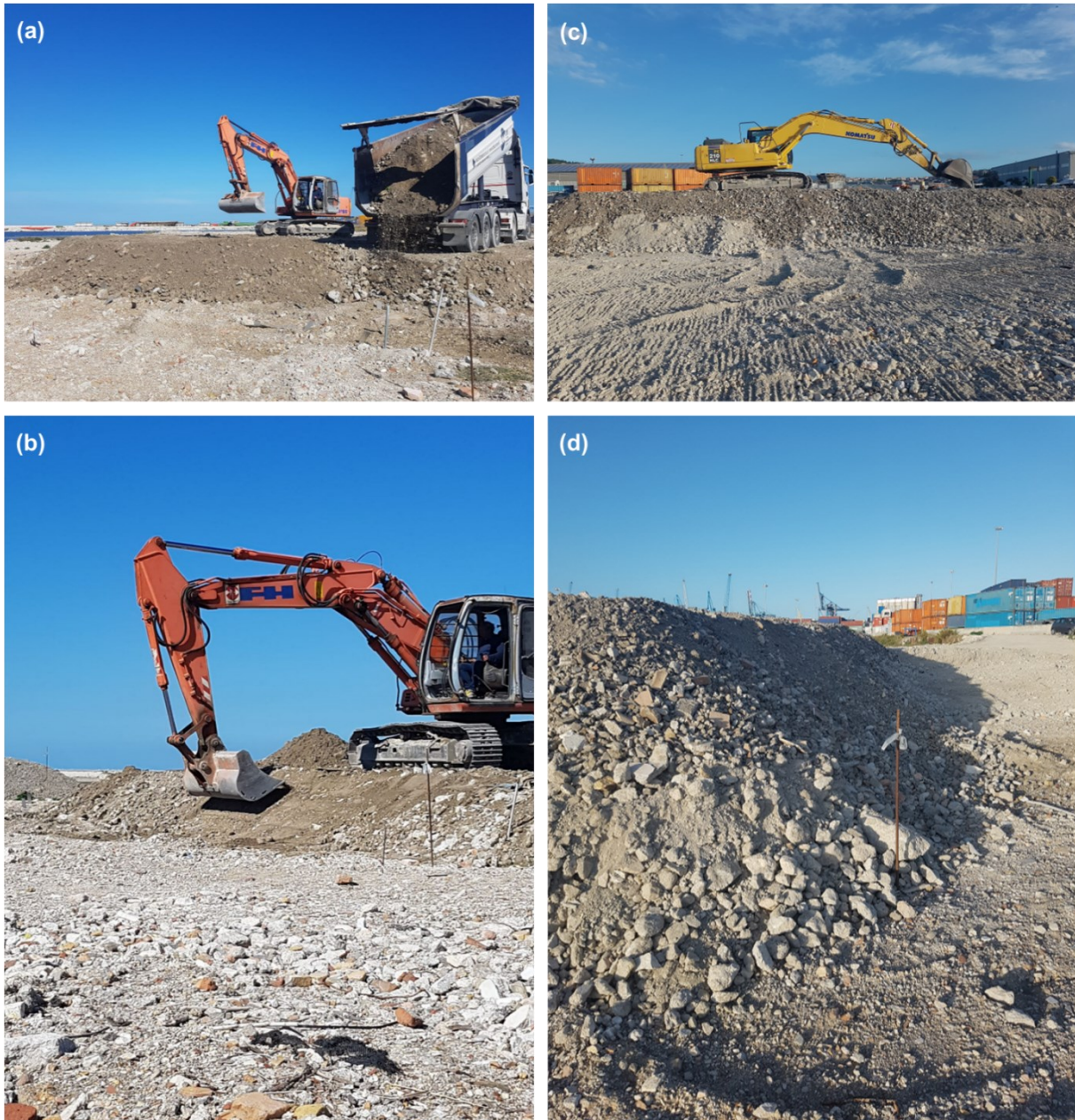
Figure 5.34. Construction of the moving embankment.
