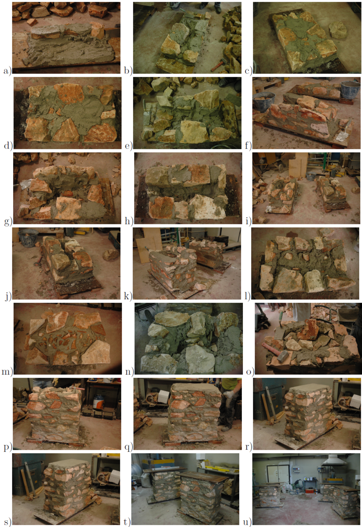
Figure 5 - "Scaglia Rossa" limestone wall matrices construction steps with the application of the double leaves' technique of the four wall matrices.
