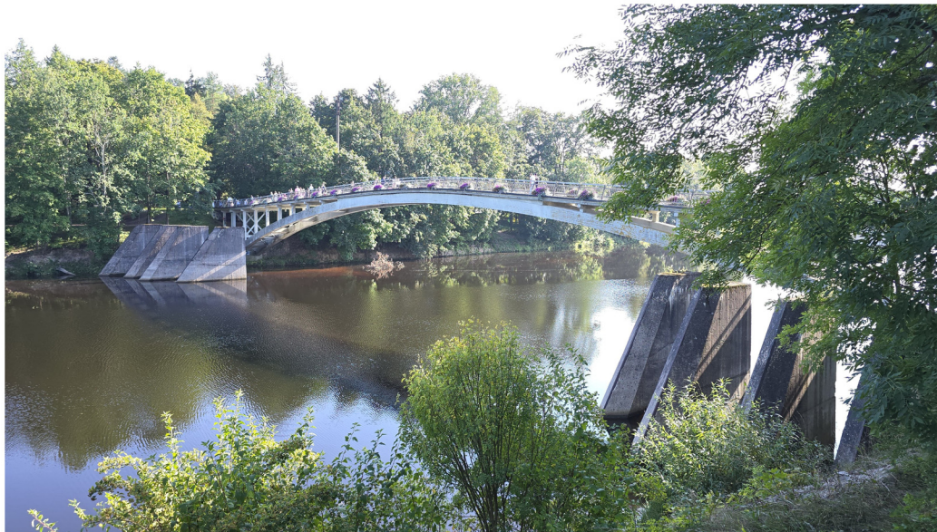
Figure 3. An example of protective measure for bridge piers, including barriers to shield against water flow and debris.
