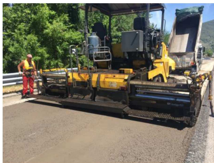
Figure 3. Laying down operations of RTM by means of a traditional road paver
