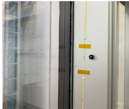
Figure 10. FBGs application on the aluminum profile for strain monitoring.
