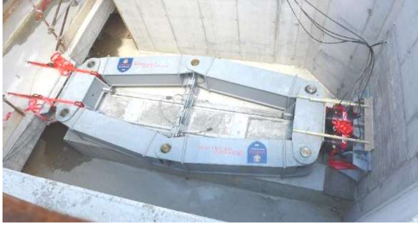
Fig. 2. Articulated steel system and reaction wall constituting the push-and-release device.
