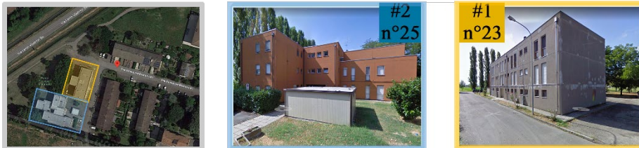
Fig. 1 The two social housing demonstrator buildings of LIFE SUPERHERO project in Reggio Emilia (Italy)
