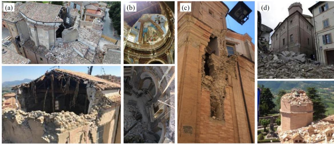
Figure 2. Earthquake damage: (a) collapse of the tiburium, (b) collapse of the dome and interior damages, (c) façade overturning mechanism, (d) collapse of the bell tower.
