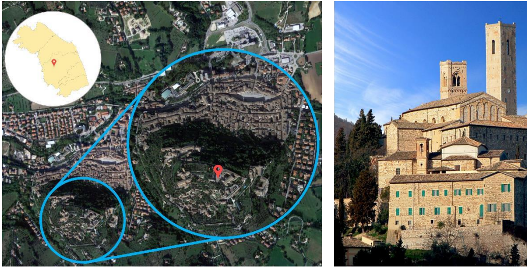
Figure 53 – Position of the Smeducci Tower (San Severino Marche, Macerata province, Italy).
