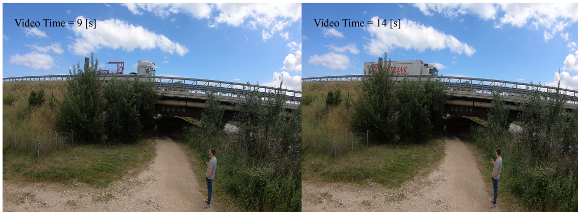
Figure 3.8: Vibrational test on the main metal beam of the bridge.
