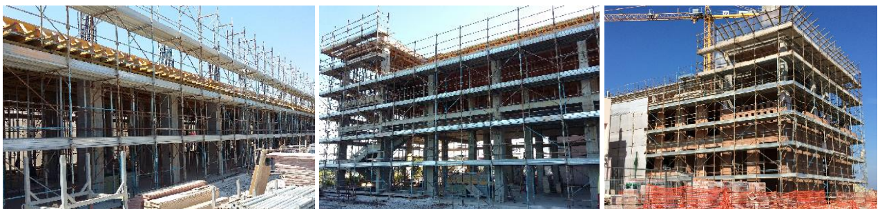
Figure 4. Pictures relevant to the construction process of the building.
