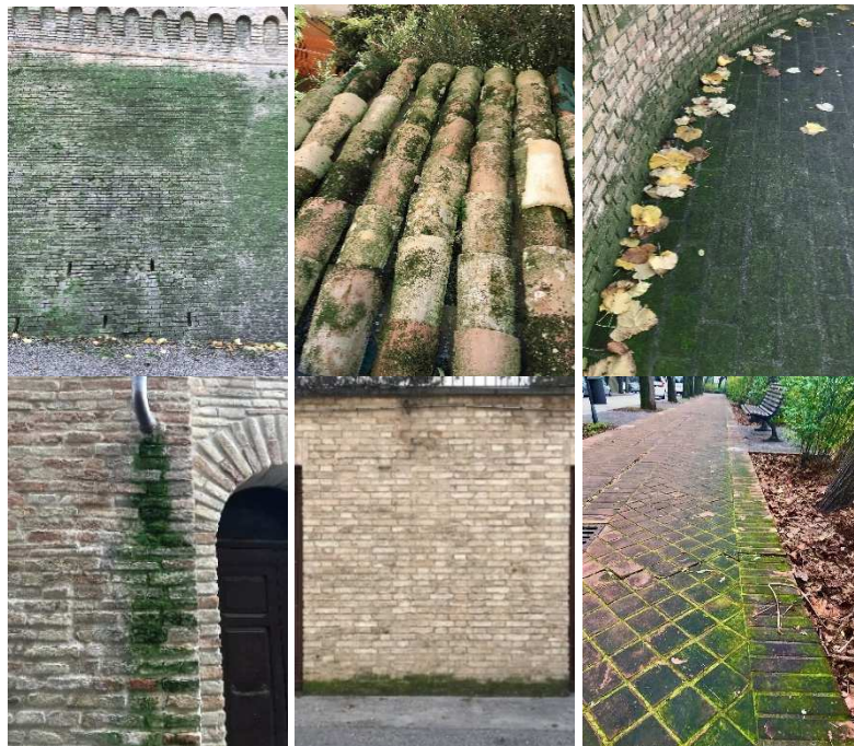
Figure 2.1 Different combination of fired bricks substrates, environmental conditions and building design details leading to algae growth.
